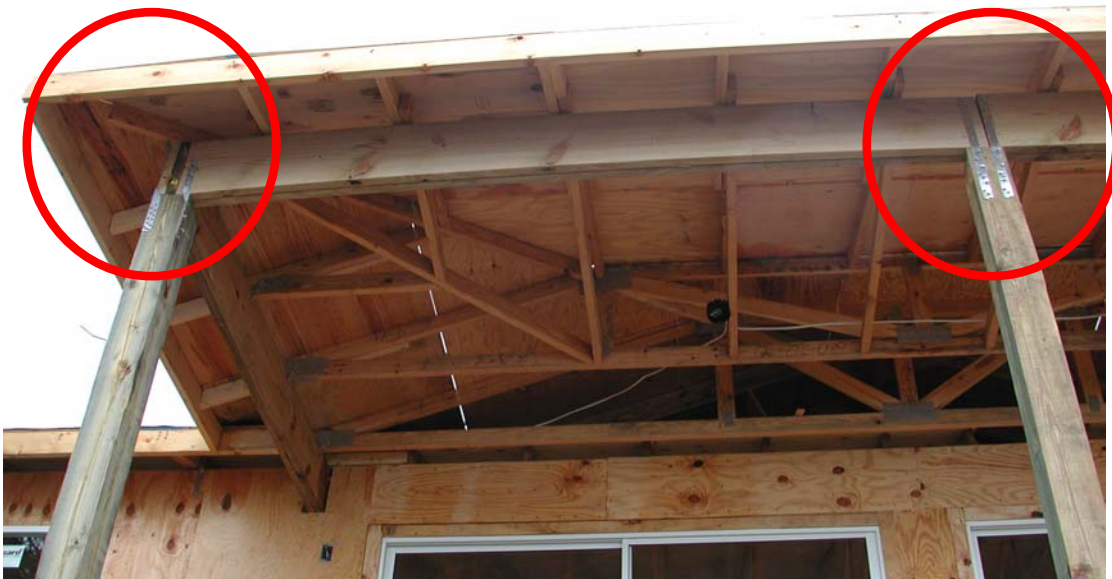
Figure 3-12: Strapping of top of porch column to supporting beam.
