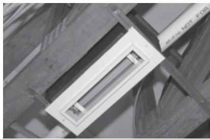
The mounting flange of the GTI Grilles will be covered by the wall and ceiling panels
